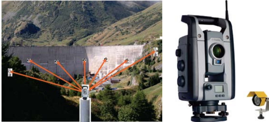
Fig 1: Total Station and prisms installation on a Dam
