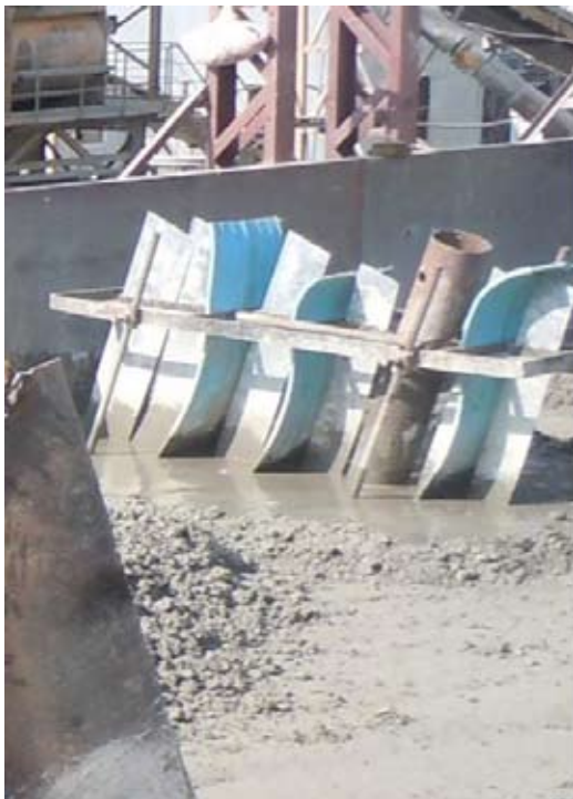
Fig. 14 : Water-stop assembly
