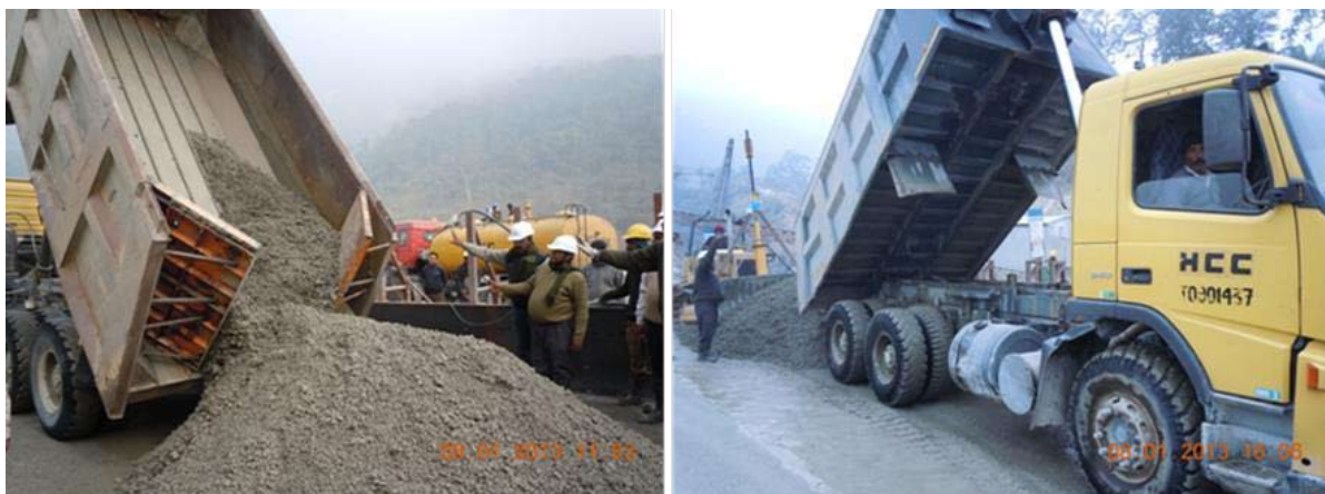
Fig. 8 : Regulated dumping of RCC from dump trucks
