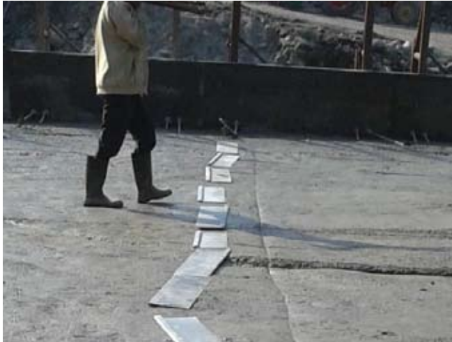
Fig. 17 : GI plates layed before insertion
