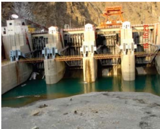
Photo 7 : Silt deposition in the stilling basin
