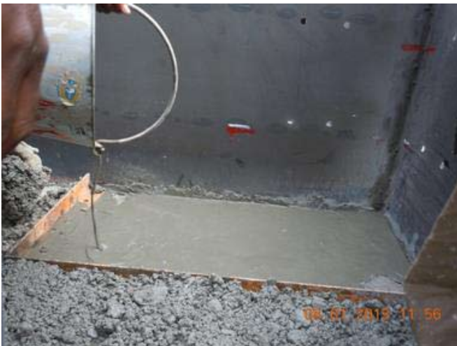
Fig. 16 : Meter stick form for preparing GEVR bund
