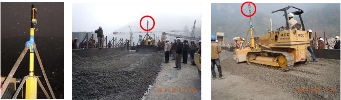
Fig. 10 : Laser guided dozing system
