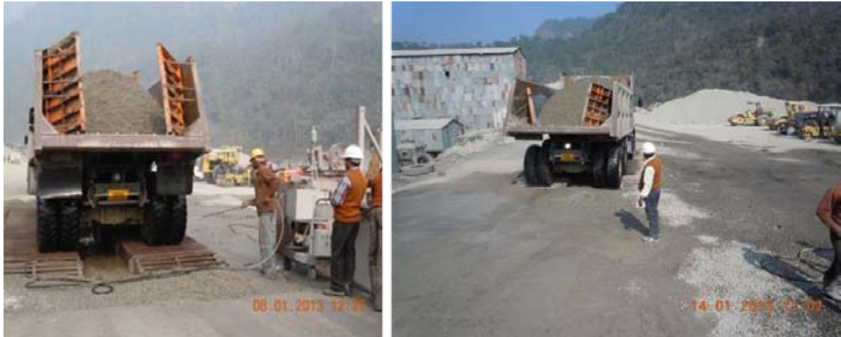
Fig. 7 : Dump trucks fitted with tapers and tire cleaning operations
