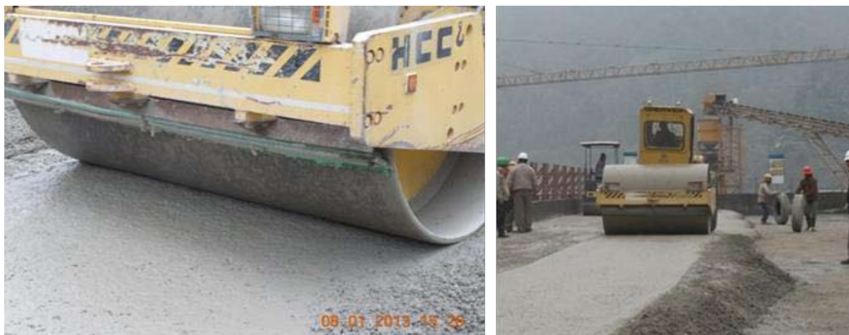
Fig. 11 : 10 MT vibratory roller under operation
