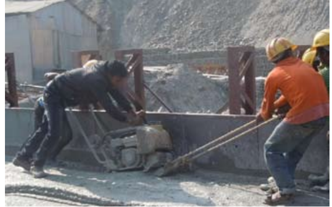
Fig. 13 : Use of plate compactor on GEVR
