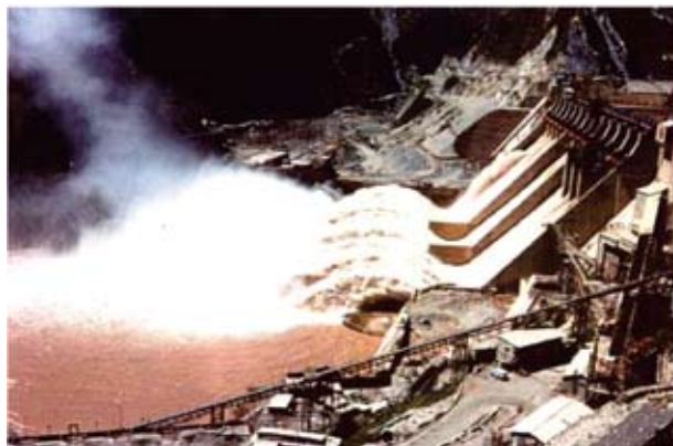
Photo 4 : Spray generation and subsequent failure of bank in Salal project
