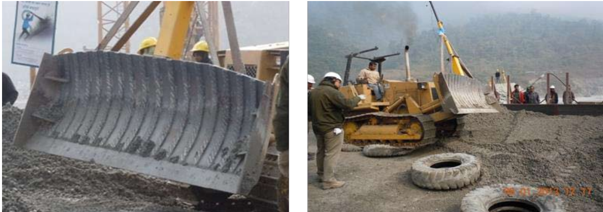
Fig. 9 : Dozers fitted with wings
