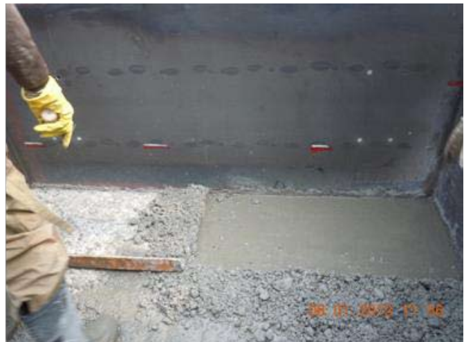
Fig. 16 : Meter stick form for preparing GEVR bund
