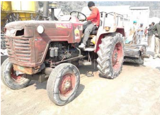
Fig. 15 : Warm joint treatment using soft brush
